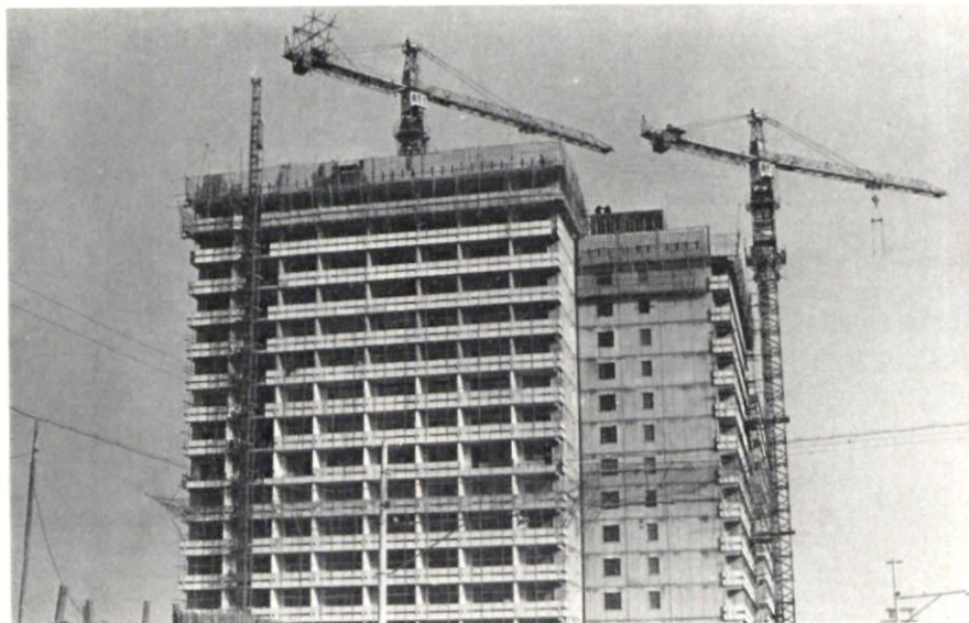
Construction in Peking, November 1976; See page 22.
