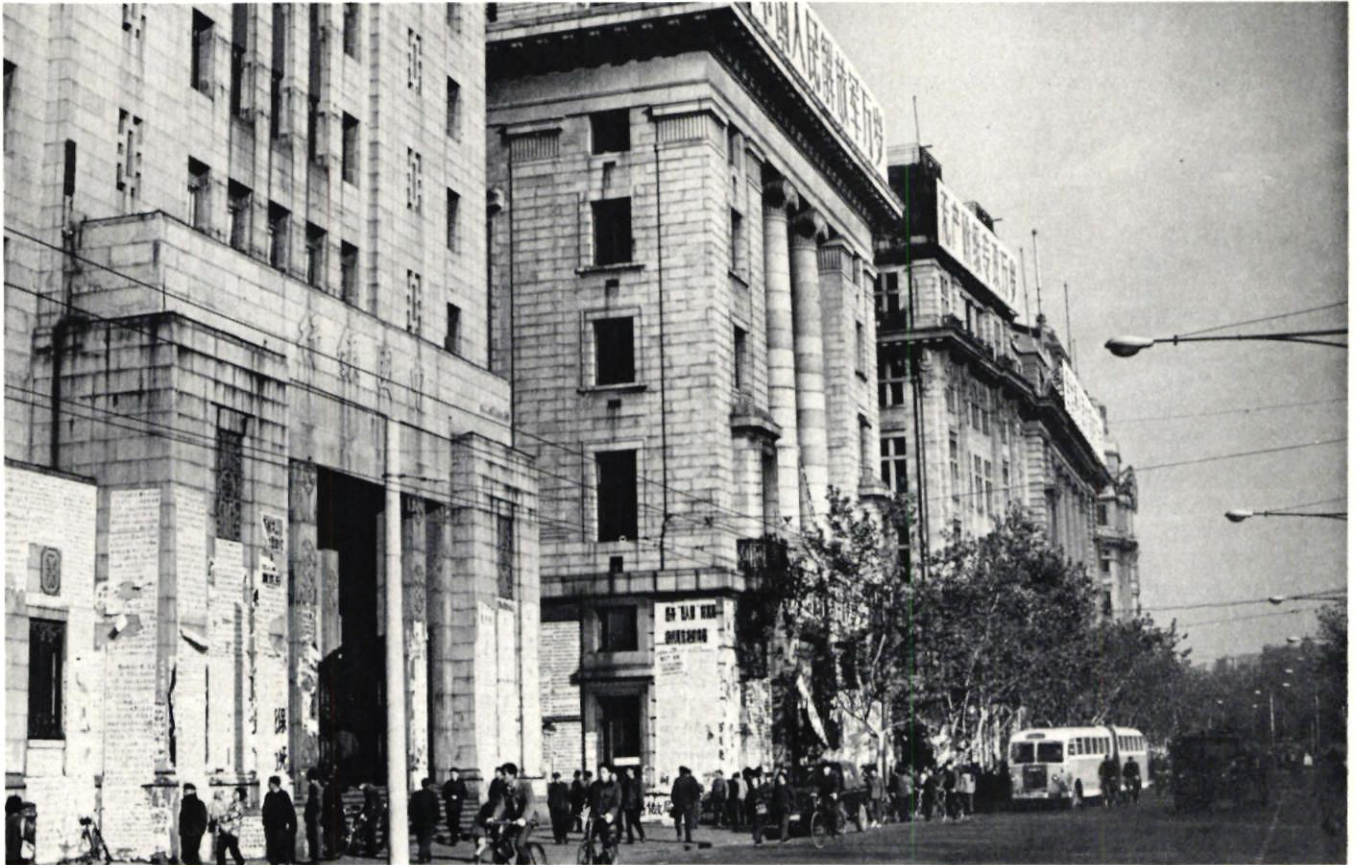
The People's Bank of China (at left) on Chungshan Road, Shanghai, November, 1976.
