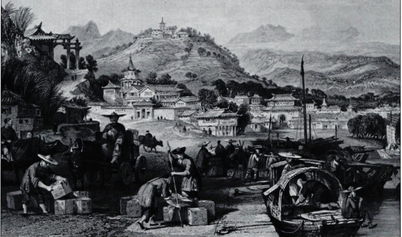
Traditional engraving of Chinese loading tea junks in the early 19th century
