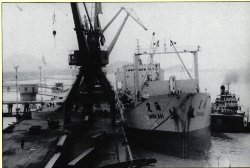
A new 10,000-tonne wharf at Nantong Port
