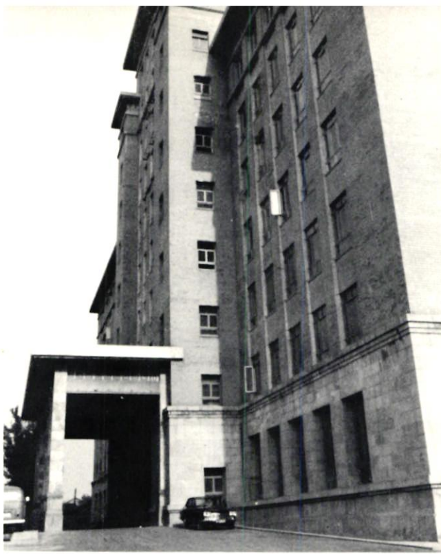
The CCPIT'S headquarters
