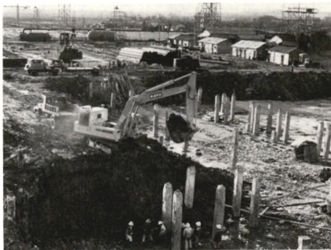
Kato backhoe at work at Shanghai site
