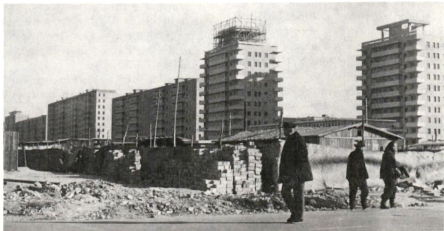
Highrise construction on outskirts of Beijing
