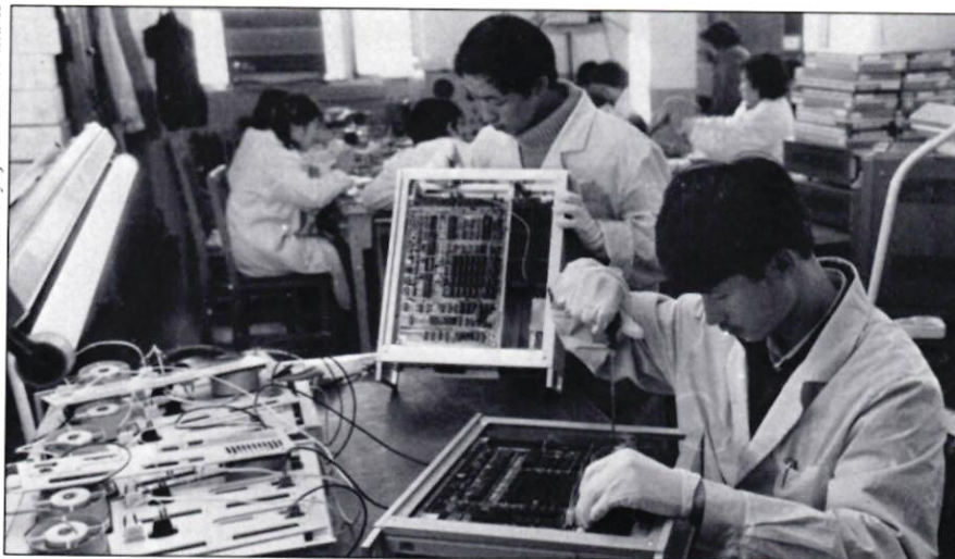
Technicians of the Beijing Institute of Electronic Computer Technology assembling BCM-III microcomputers.
