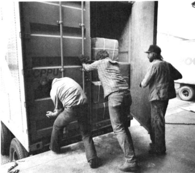
Combining traditional breakbulk methods and modern intermodal shipping: cargo is transferred to piggyback railroad trailers.
