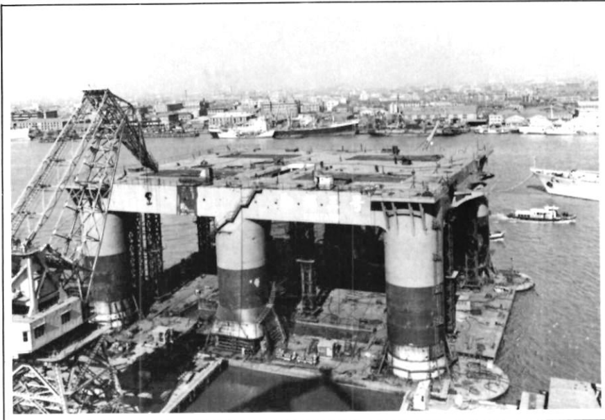
The Kantan III, China's first semisubmersible, is one of five offshore rigs under construction in Chinese yards.
