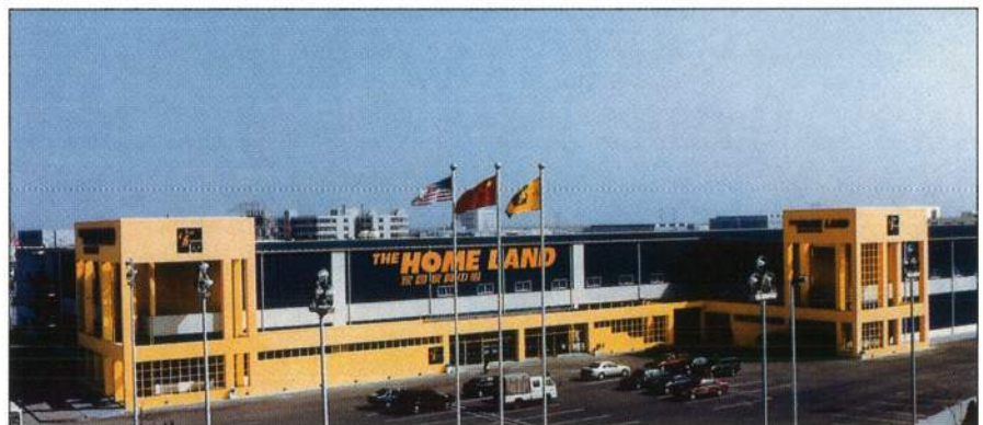
The Cris Group and Cris Real Estate Company Ltd. customized Butler's Widespan structure for its retail furniture store in Tianjin. The building was shipped by truck from Butler (Shanghai). photo courtesy of Butler Manufacturing Co.
