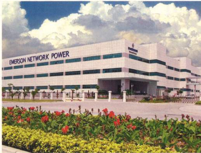
Emerson Network Power, Shenzhen. Courtesy of Emerson.
