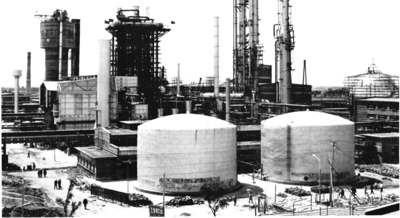
A Toyo ammonia/urea fertilizer plant in Chengtu: Chinese endusers have been trained in Japan to operate plant.
